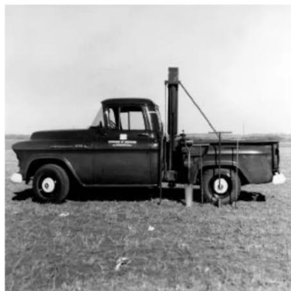
Example of a power probe truck and field hand tools used in the 1950's by Nebraska soil scientists. This unit used by Dean DaMoude, Cuming County, 1957.
