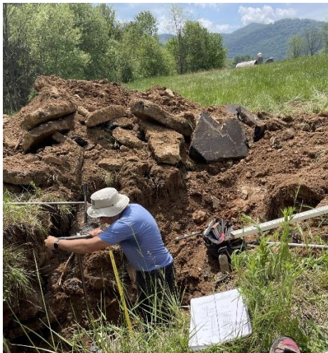
Concrete Fill Material in Basin 1
